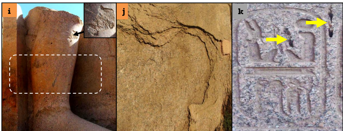
Figure.1.Deterioration features of granite stoneworks at Karnak temples; (i) Staining and contour scaling. (j) Exfoliation. (k) Birds droppings.
