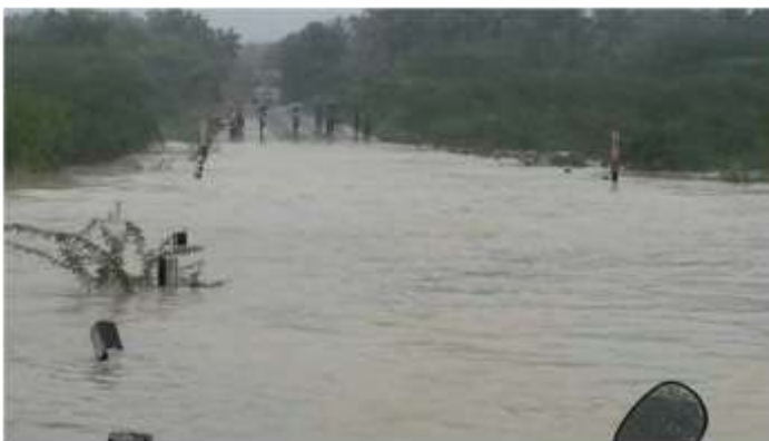
Fig. 2 Flooded Maninagar causeway
