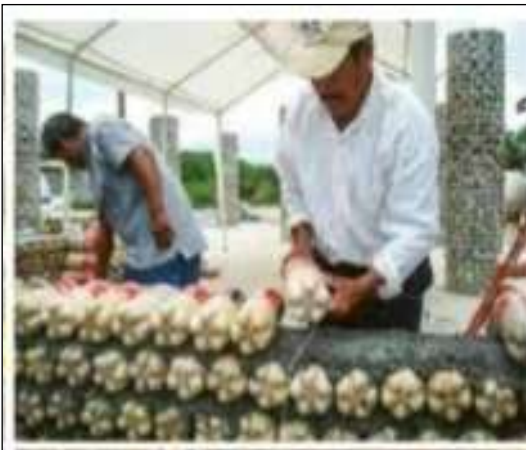
Fig. 1 – Houses constructed using PET bottles
