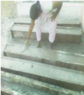
Fig.5 Casting of Beams
