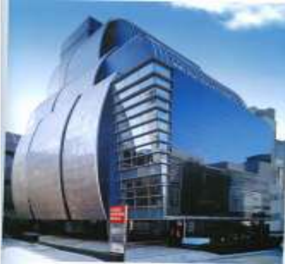
Figure 7.Hong Kong Science Building with photoelectric facades.
