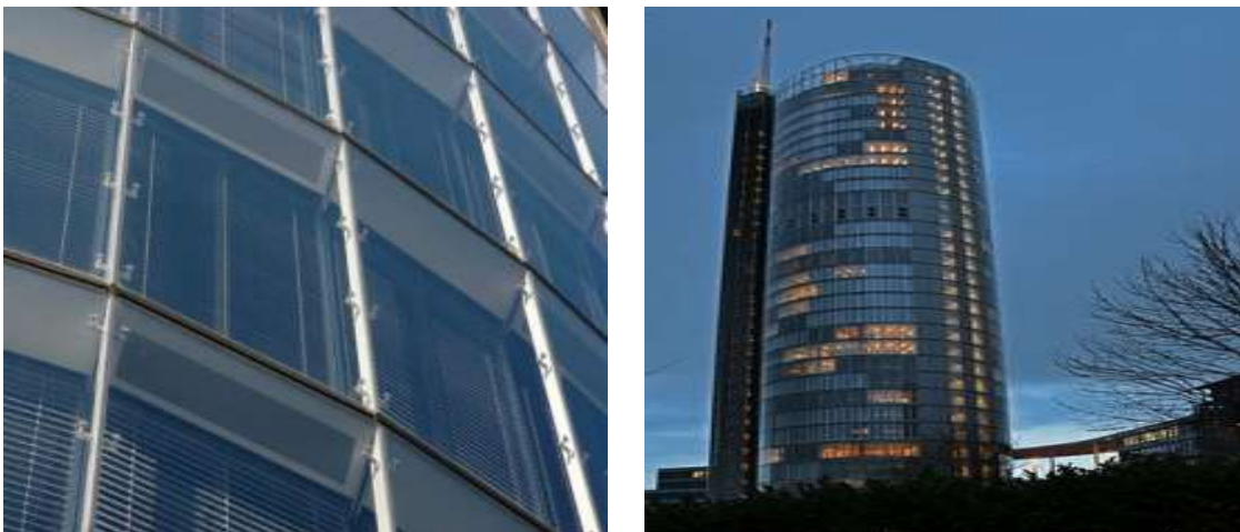
Figure 6. Mechanical shading techniques used in aluminum and glass curtains in the building.
