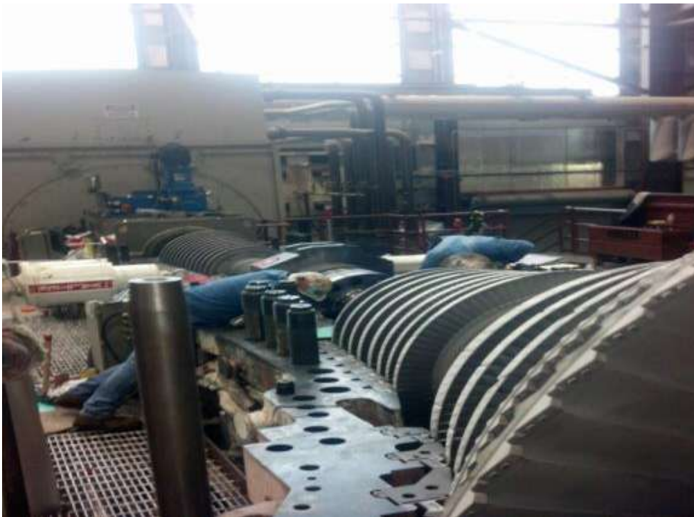
Figure 6.Erection of Turbine
