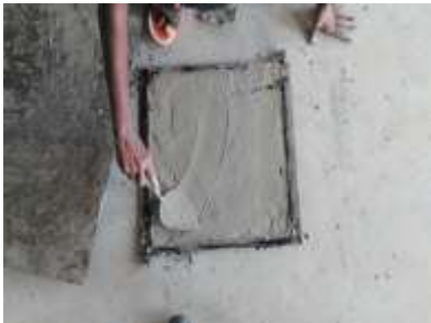
Fig . 1 Casting of the specimen
