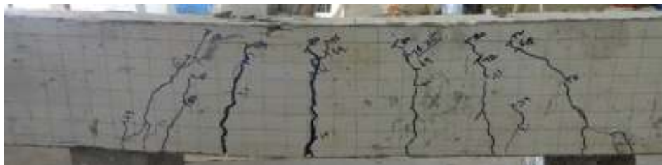
Fig.4 Crack pattern of control beam
