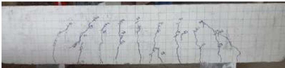
Fig.5 Crack pattern of W-1
