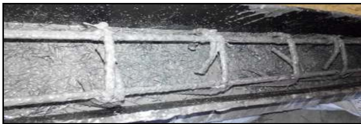
Fig.2. Casting of SIFCON beam
