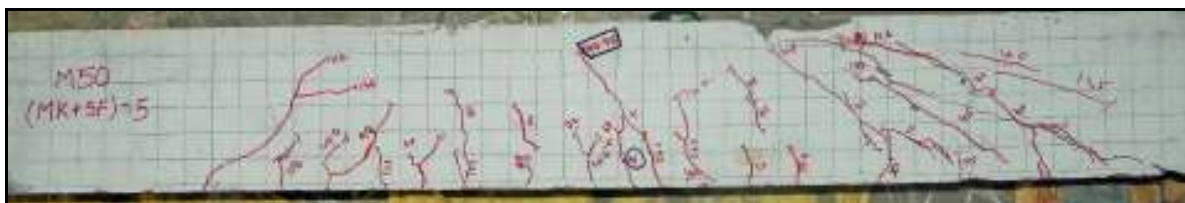
d. Crack pattern for M50 optimum mix (MK+SF)-5 beam
