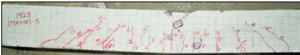
b. Crack pattern for M25 optimum mix (MK+SF)-5 beam
