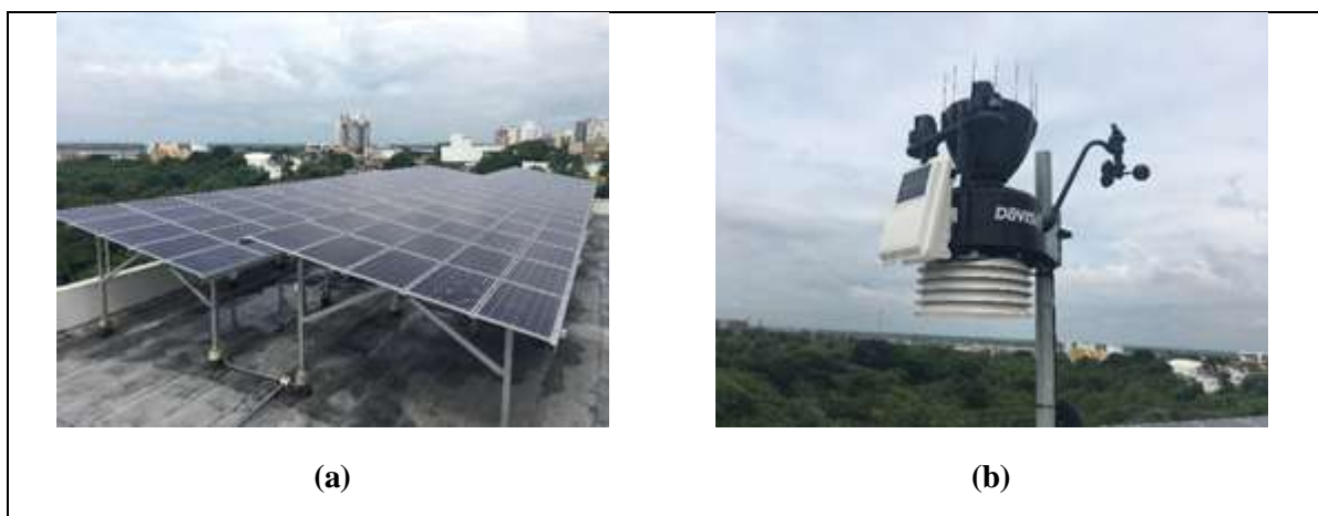
Fig. 1. (a) PV solar modules array; (b) Weather station.
