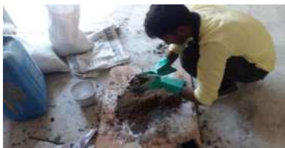
Mixing of raw materials
