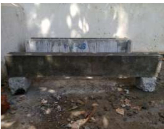
Fig 4.2. Casting of Beams
