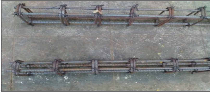
Figure 1. Reinforcement of the beam
