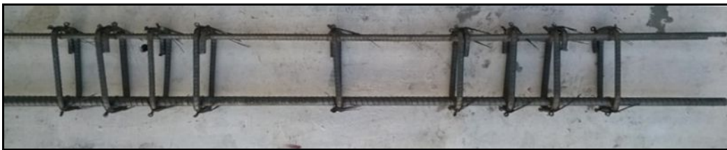
Fig.1 Reinforcement setup of B-2
