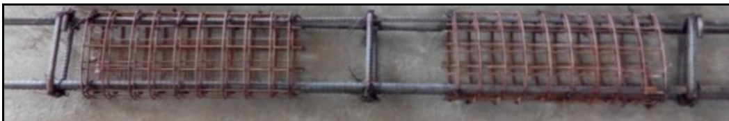
Fig.3 Reinforcement setup of B-3
