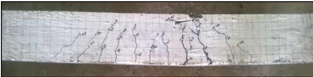
Fig.7 Crack pattern of B-2
