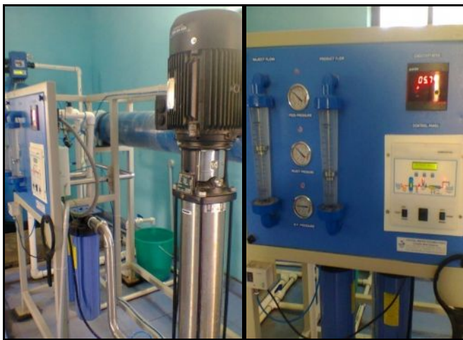
Figure 1. Photographs of Reverse osmosis plant
